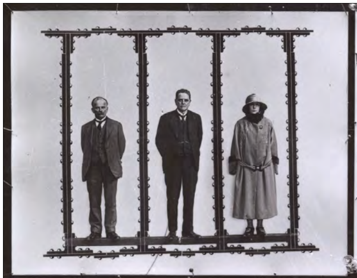
John Bradfield, R.T.Ball and Miss Butler, all appearing to stand within a cross section of the lower chord of the Sydney Harbour Bridge.
