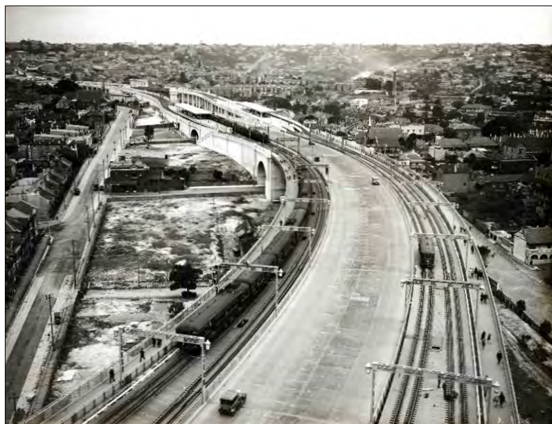
The North Sydney bridge approaches, photographed from the north-east pylon on 18th April 1932. Both train & tram station roofs at Milson's Point are visible, with trains in both directions, a solitary tram travelling north & many walkers.
