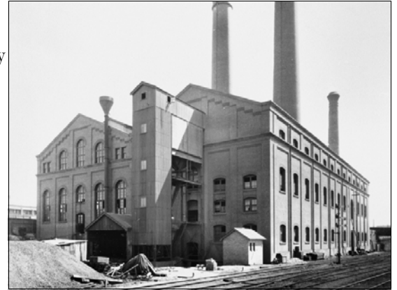
The back of the Power Station in c.1905, viewed from south-east. The boiler house is on the right, the engine room & Turbine Hall at left. Photo: Powerhouse Museum.
