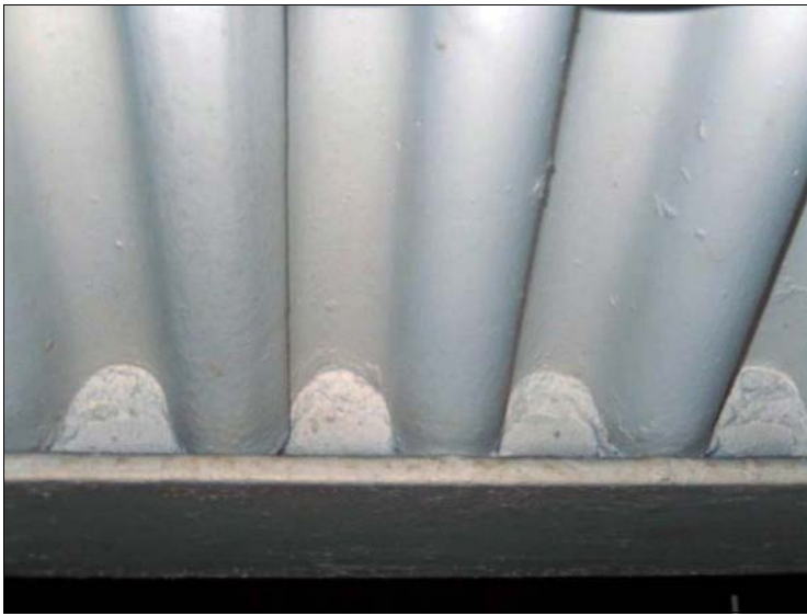
Australian Museum, College Street, Sydney, Traegerwellblech ceiling in the Vernon wing: Photo: Peter Phillips.
