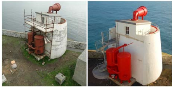
The Foghorn, before and after repair & restoration. Images from IMechE website.
