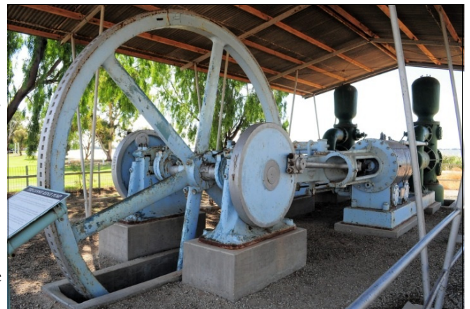
The Cannie Ridge Pumping engine in its shed on the shores of Lake Boga, which can be glimpsed in the background. Image: O. Peake.
