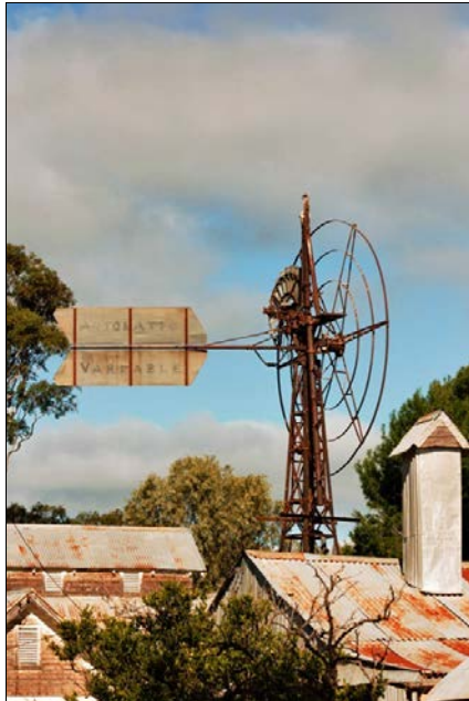
Above: Fortescue variable stroke windmill. Image: T. Glastonbury.
