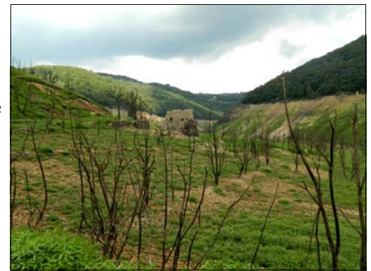
The empty dam in 2015, with a ruin (perhaps a former mill?) in the background. Photo: Merv Lindsay.
