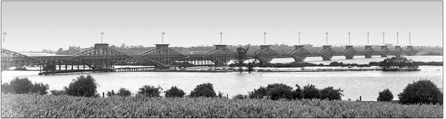
The Barwon Sewer Aqueduct at completion, during a flood on the Barwon River.
