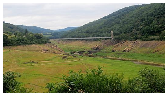
A new bridge overlies an ancient bridge. Photo: Merv Lindsay.
