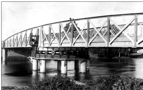
Swing Bridge, near Sale, designed by engineer John Grainger - built 1883. Image: Sale Historical Society.
