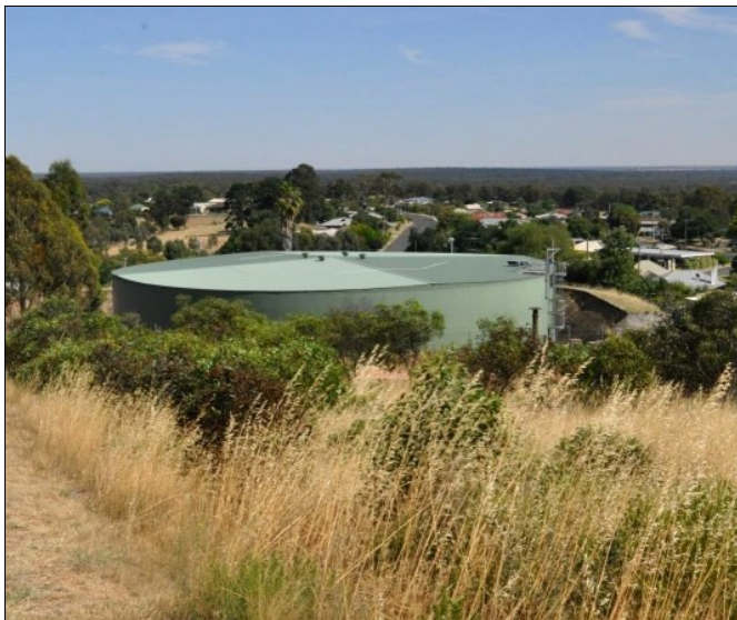
A modern, roofed water storage tank built inside the original open topped circular No.1 reservoir on Big Hill in Stawell. Source: Owen Peake 2013
