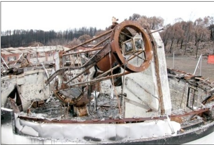
Two views of what was left of the Great Melbourne Telescope after the 2003 bushfire at Mt Stromlo Observatory.
