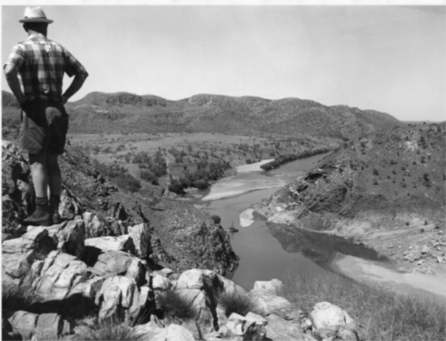
August 1968 Abutment of the Ord River Dam
