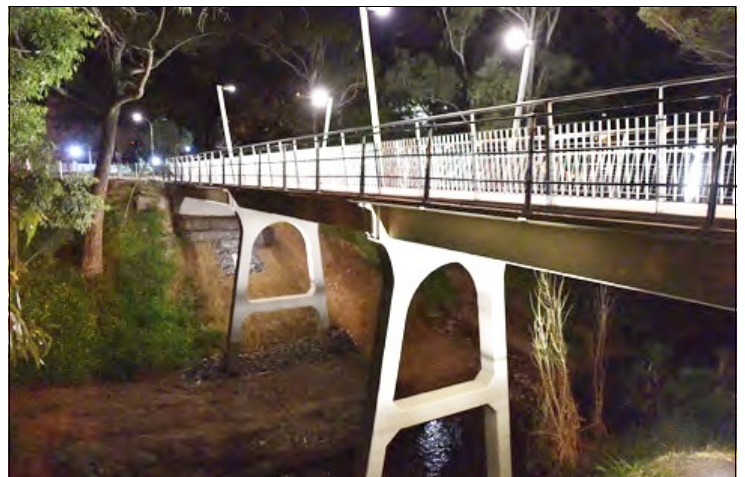
Sir William Goodman Bridge after restoration.
