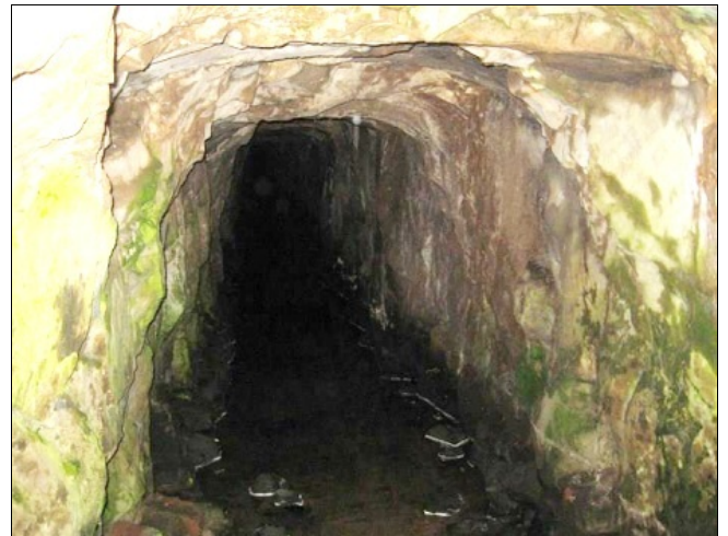
Inside the water supply tunnel in 1979 Photo: Miles Pierce
