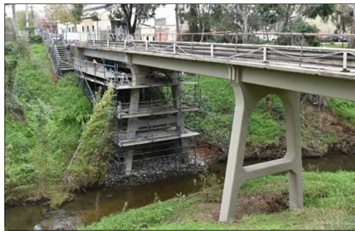
The Sir William Goodman Bridge during restoration. Photo - John Woodside.
