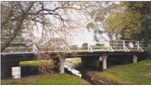
St Kilda Street Bridge - west side. 1997 photo by Lesley Alves.
