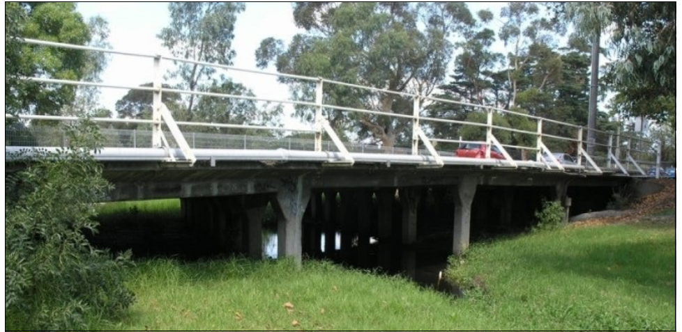
St Kilda Street Bridge photographed from the west side.
