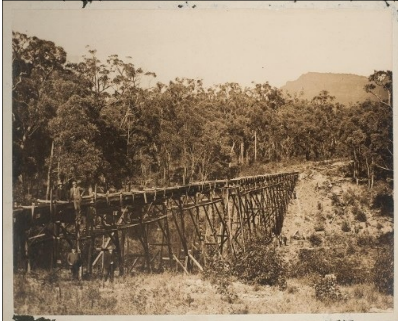
An original timber trestle viaduct carrying the flume across a creek. Source: Unknown.
