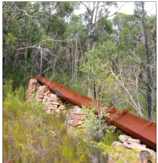
Steel flume carried on stone pillars, photographed in February 2014. Source: Flickr - Rf-toaster, Stawell Water Supply Walk 2014 - img7256
