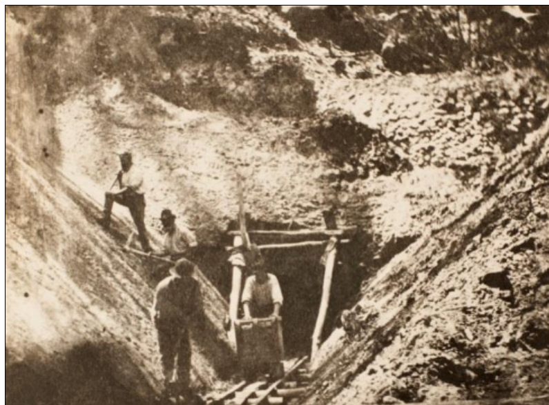
Digging the eastern end of the tunnel under the Mt William Range. Source: Public Records Office Victoria.
