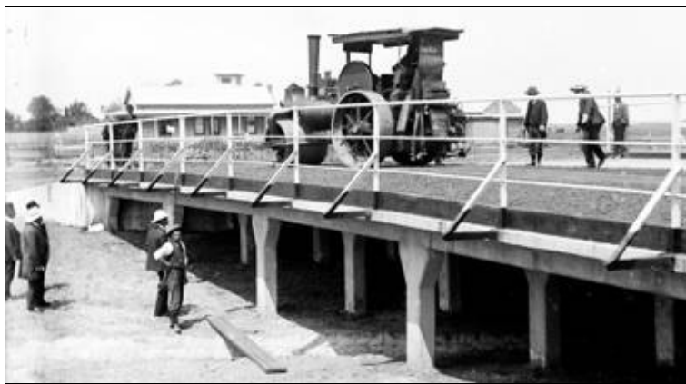
St Kilda St Bridge Load Test, 20 th November 1905. Source - Melb University Archives.
