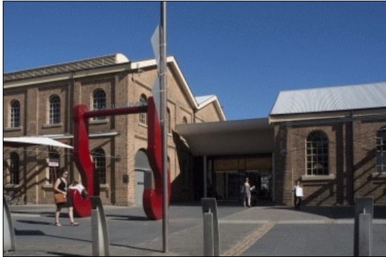
Honeysuckle Point Boiler Shop (L) and Blacksmiths' Shop (R). The linking structure is new and was built for the Museum.
