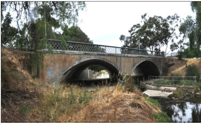
King's Bridge, Bendigo.
