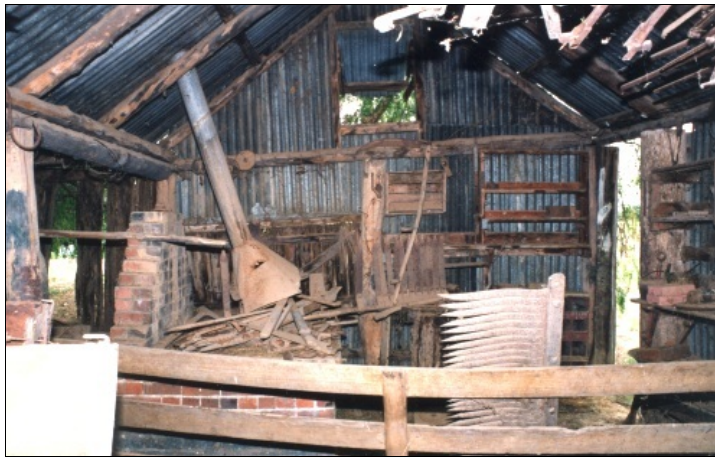
Blacksmith Shop interior & Forge 'as found'
