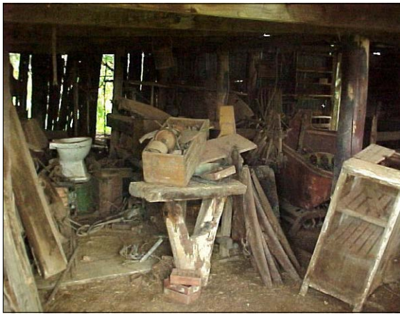
Blacksmith Shop interior 'as found'
