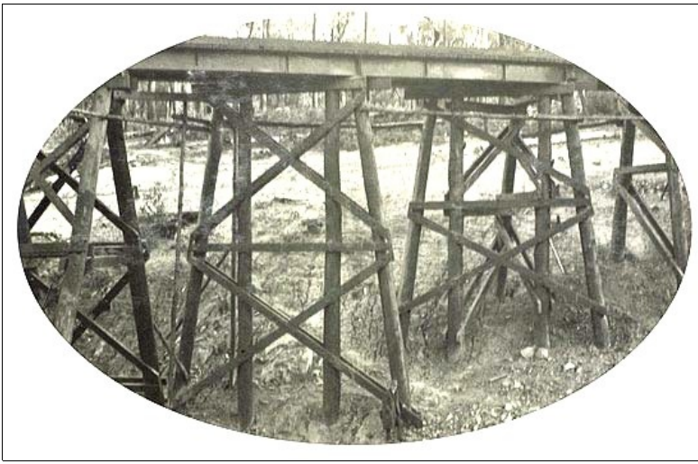
Right: The Wairewa Road O'Grady's Creek trestle bridge under construction in 1914-1915. Timber trestles/piers and cross beams are complete and the wrought-iron rivetted girders are set on the cross beams but not yet fixed in place. These girders are said to have been recycled from a bridge on the North East line to Wodonga – probably the bridge over the Broken River at Benalla, which was rebuilt with larger steel girders at about the same time. The recycling is typical of Kernot, to whom economy and keeping costs down was extremely important. From Charles H Perrin Album.
