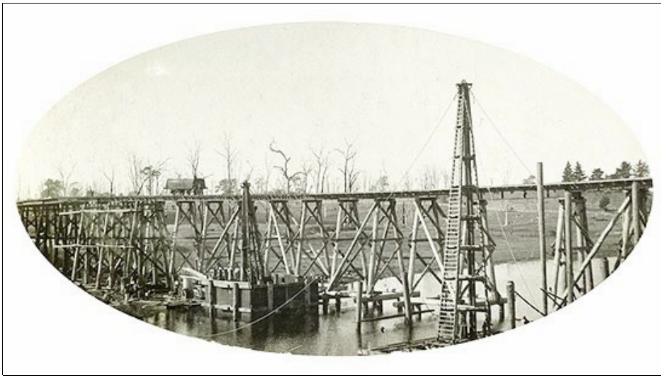
The Nicholson River crossing in 1915. Note the wagon on the temporary trestle bridge, the coffer dam for Pier 4 at left, and the pile driving derrick at right. Source – Charles H Perrin Album.
