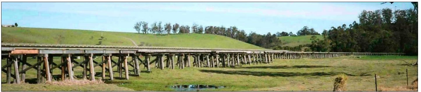
The Snowy River flood-plain railway viaduct at Orbost in 2000.
