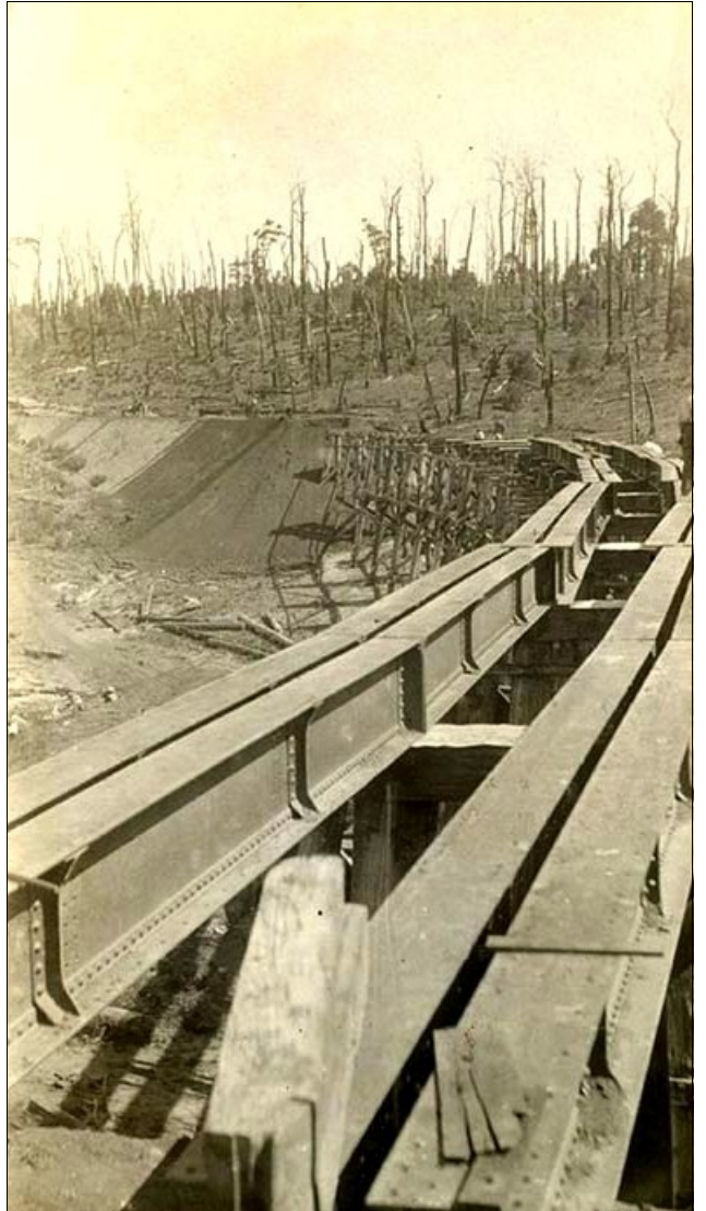
Right: The Wairewa Road O'Grady's Creek trestle bridge under construction in 1914-1915. Timber trestles/piers and cross beams are complete and the wrought-iron rivetted girders are set on the cross beams but not yet fixed in place. These girders are said to have been recycled from a bridge on the North East line to Wodonga – probably the bridge over the Broken River at Benalla, which was rebuilt with larger steel girders at about the same time. The recycling is typical of Kernot, to whom economy and keeping costs down was extremely important. From Charles H Perrin Album.
