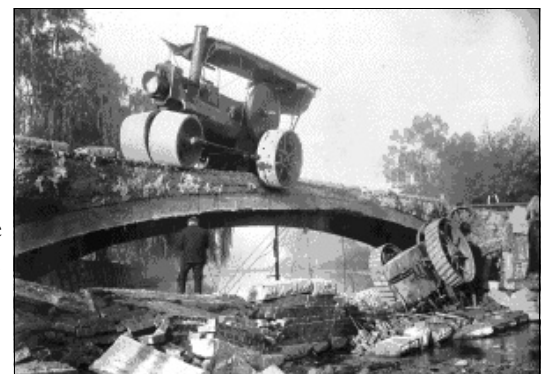
King's Bridge after testing failure.
