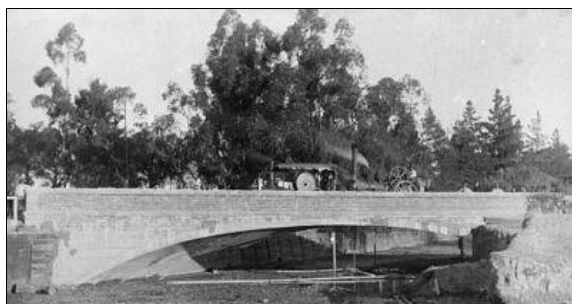
King's Bridge under test before failure
