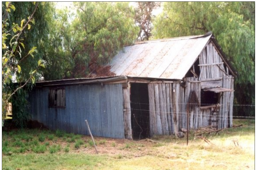
Blacksmith Shop viewed from SW showing the skillion built on the west wall
